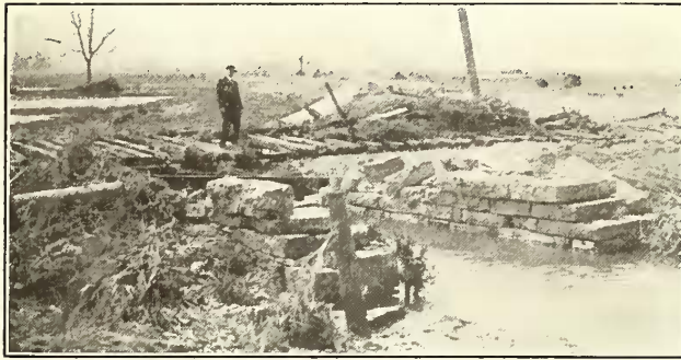
Ohio Flood—Washed-Out Culvert on Ohio Electric Railway
